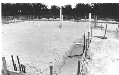
The "Foundation" for this slab home is the "turned-down" portion of the slab at the perimeter. Notice the plumbing pipes which will poke up through the slab.
