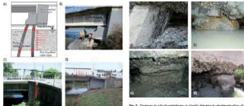
Fig. 5. Damage to abutments: a) sketch of lateral spreading forces acting on abutments and foundations; b) buckled abutments of Bridge Street Bridge (photo: M. Branshaw); c) buckled abutments of Fitzgerald Avenue Bridge (courtesy of DPUS International Ltd); d) damage to abutments of Avondale Road Bridge (courtesy of DPUS International Ltd)
