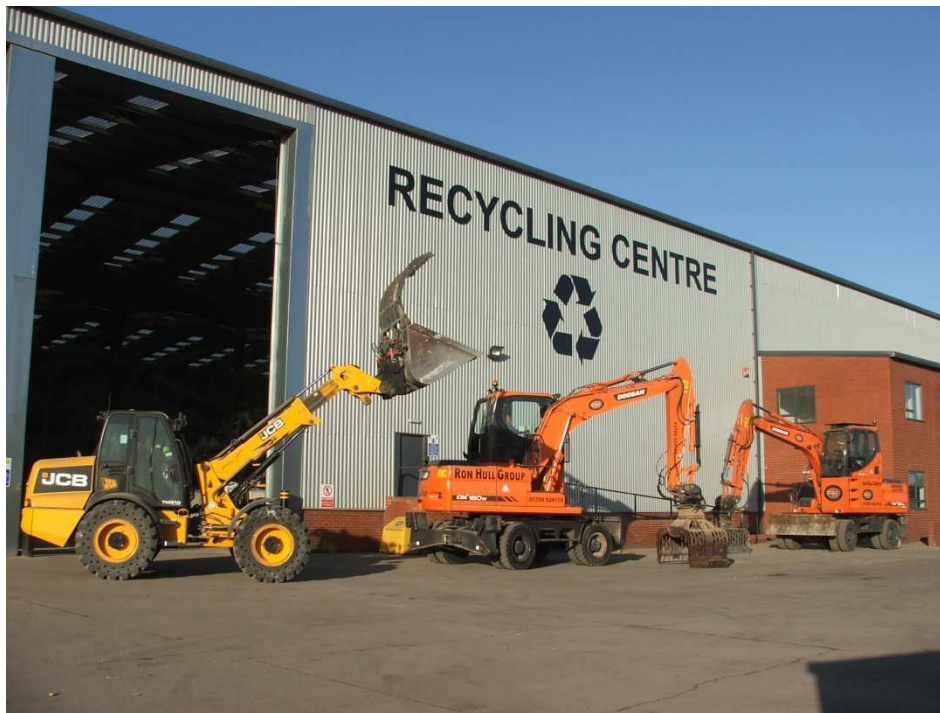
Pic 19. A Recycling Plant
