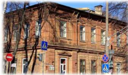
Figure 3. House of V. M. Lemke in Kanatnaya Street
