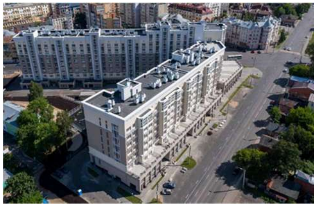
Figure 1. Residential complex «Simfoniya Nizhnego»
