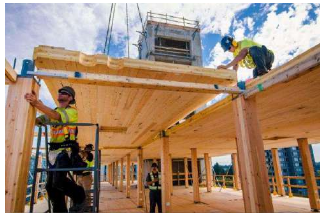
Figure 5. Dormitory in Canada
