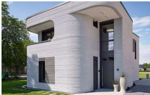
Figure 2. Two-storey mansion in Beckum, Germany
