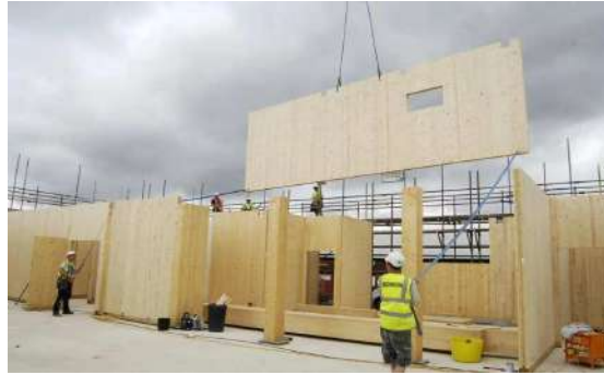
Figure 3. CLT – panel mounting
