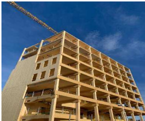
Figure 4. Office building in Norway
