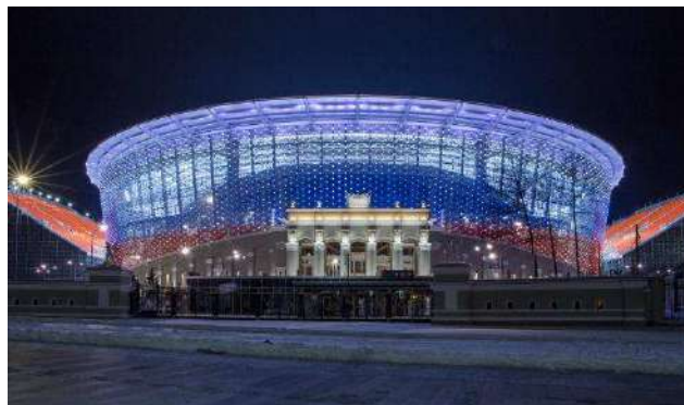
Figure 2. Media facade of the Yekaterinburg Arena stadium
