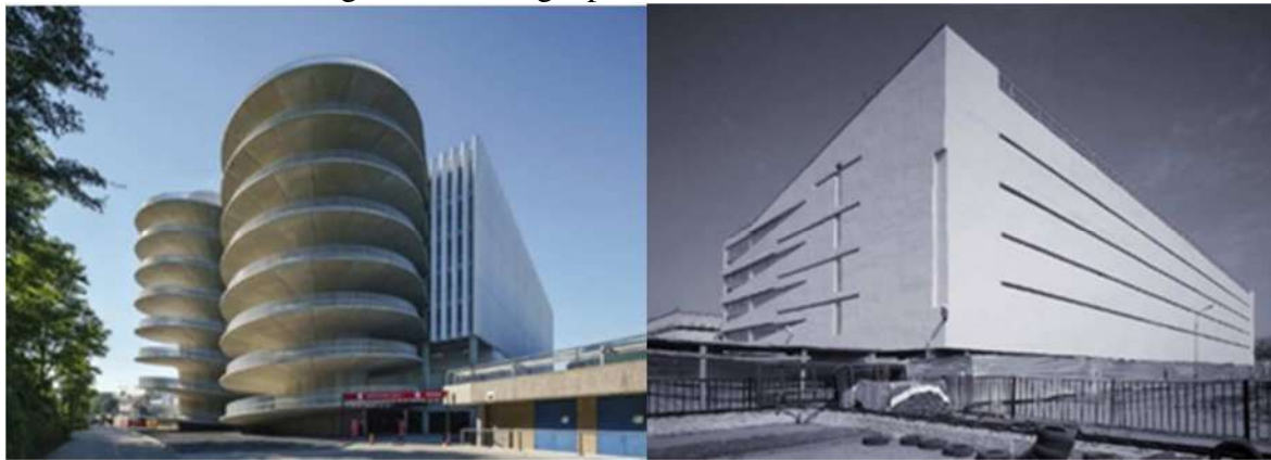
Figure 3. Parking RAI aux Pays-Bas
