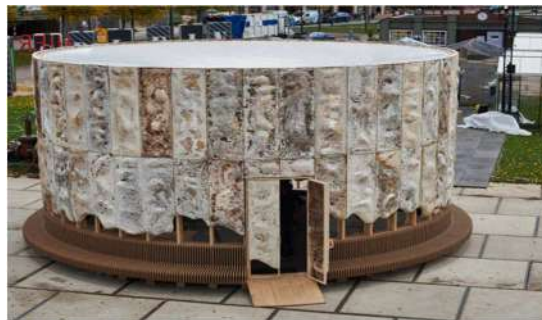
Figure 1. Biodegradable pavilion made of mushroom mycelium
