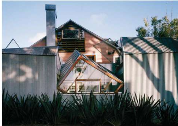
Figure 1. Residence in Santa Monica
