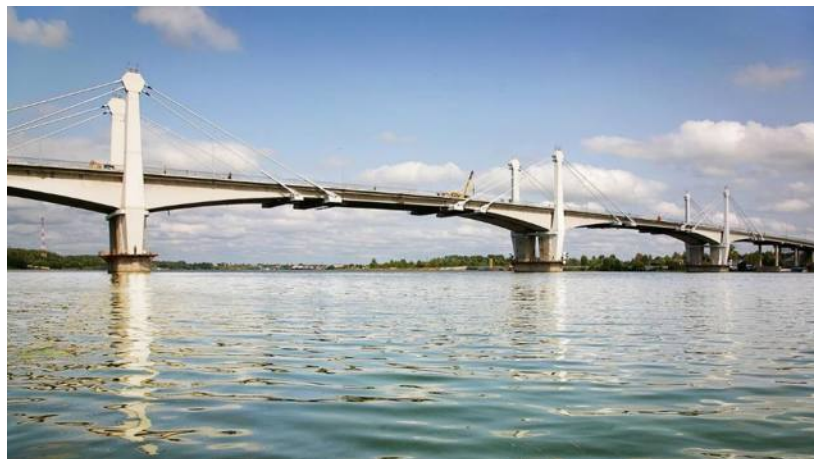
Fig. 1. Structure of Krimsky Bridge
