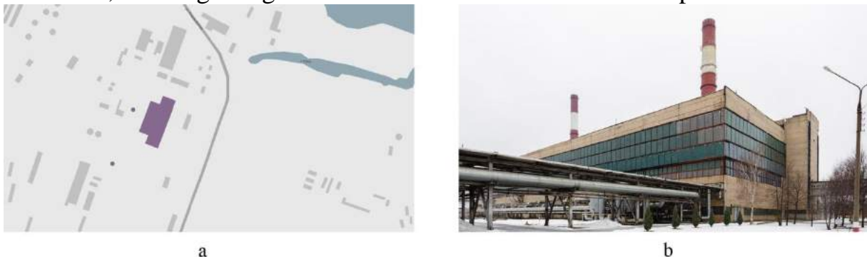
Fig. 3. Thermal power Plant, Sormovo, Nizhny Novgorod: a) general plan; b) general form
