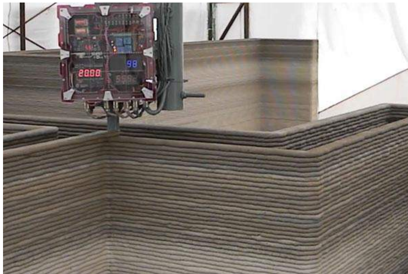
Fig.2. The process of printing the internal and external walls
