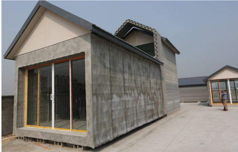
Fig.1. A house built from debris
