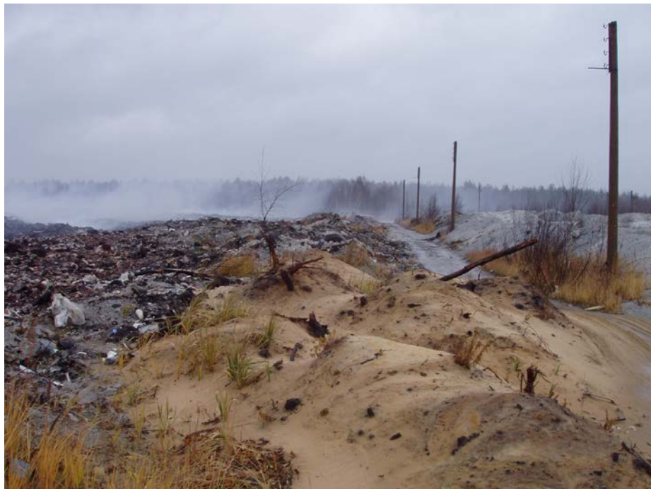
Fig. 1.19 Non-operational industrial waste disposal site, where wastes are continued to be dumped daily
