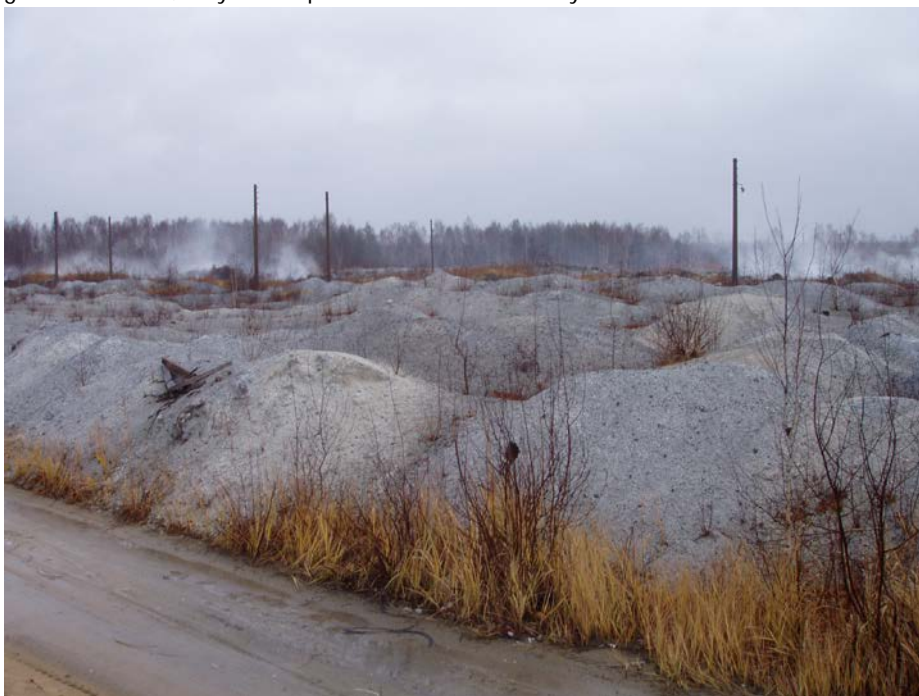
Fig. 1.20 Ash-and-slime wastes of the Igumovo heat power plant on the karstified territory in the valley of the Oka river
