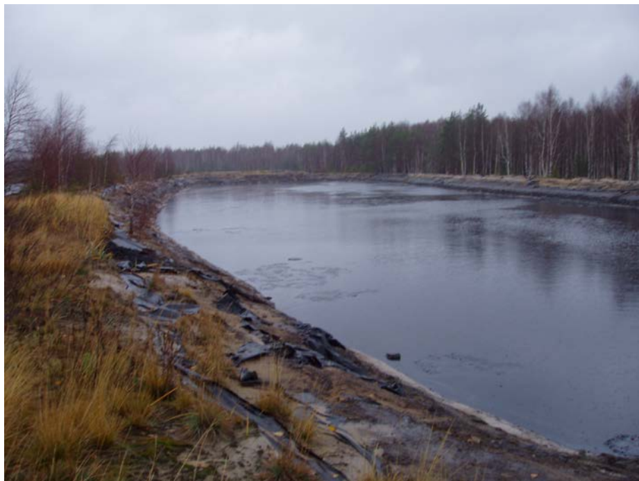
Fig. 1.8 The pond is filled with wastes to a depth of 2.5 m. The surface is covered with black oily liquid
